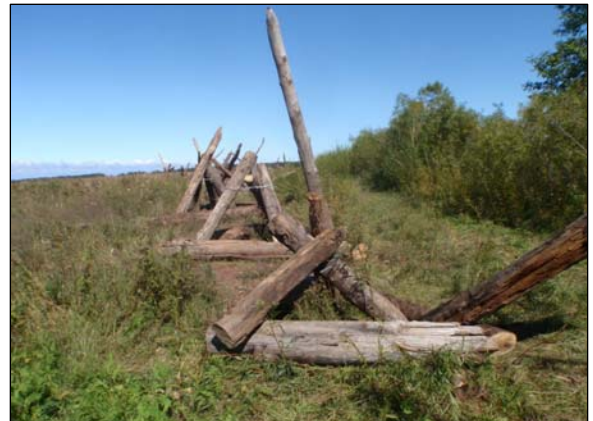
Aquatic habitat structures are built from old-growth pine.
